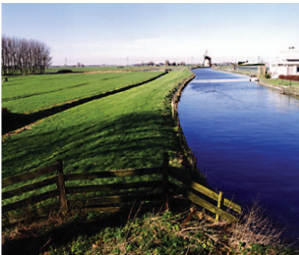
Figure 3. Deep polder (reclaimed land, green grassland at left) in the western part of the Netherlands.
